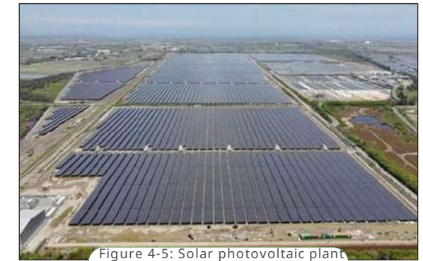
Figure 4-5: Solar photovoltaic plant in Qigu, Tainan
