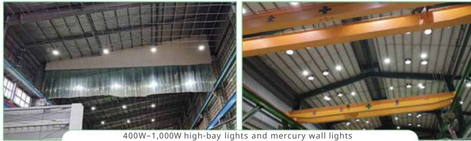
400W-1,000W high-bay lights and mercury wall lights replaced with 150W-240W LED lights
