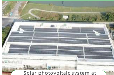
Solar photovoltaic system at Nanke Plant
