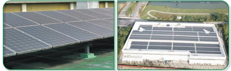
Self-Built Solar Power Device - Energy Installation in Linko North Plant and Nanke South Plant
