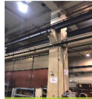
400W old lights to retire & change to 150W LED
